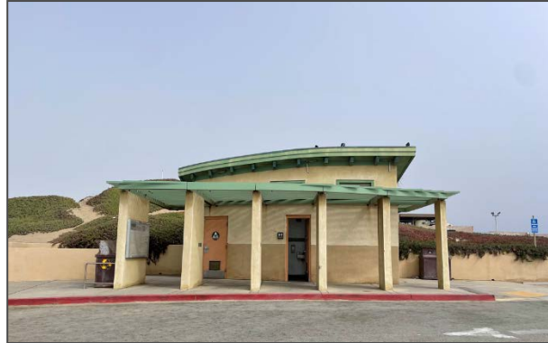
Restroom at Marina State Beach Parking Lot Photo credit: EMC Planning Group
